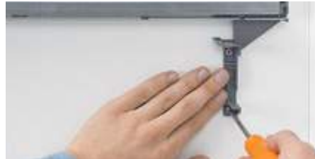
2. Position bracket profile attachment and screw on
